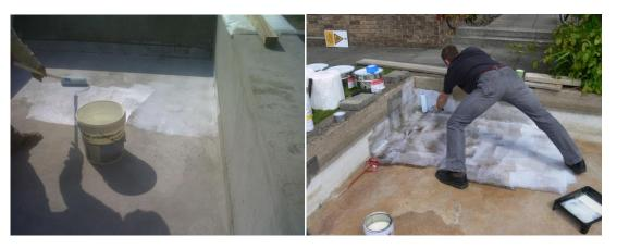
2- Reinforcement of singular points: cracks, joints, corners, passing pipes, drains...Apply a first thin layer of Impermax ST/QC and reinforce with the geotextile GEOMAX. The Rayston Fiber 150 grams/m² or the self adhesive strip Butyl Tex could also be used.
