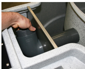
Figure 17.2 - Move 90° to by-pass
